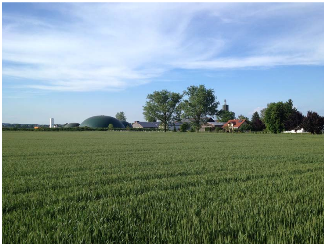
Biogasanlage in Oberindling
